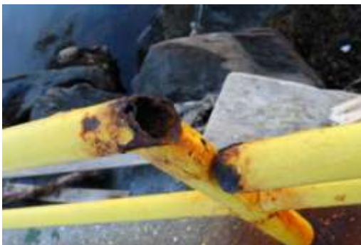
Failure due to corrosion Figure 1
