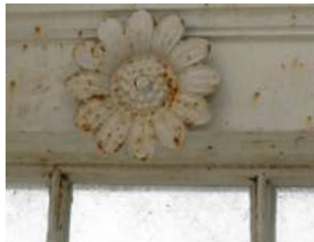
Pinhole Corrosion Figure 7
