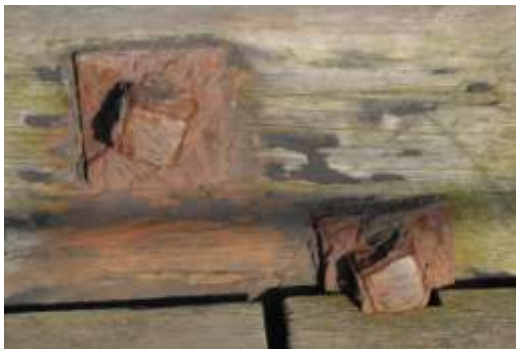
General Corrosion Figure 3
