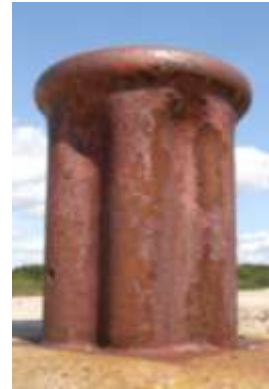
Corrosion Allowance Figure 4
