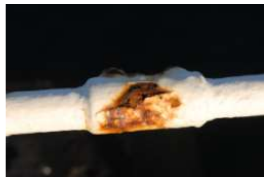
Severe coating breakdown Figure 8
