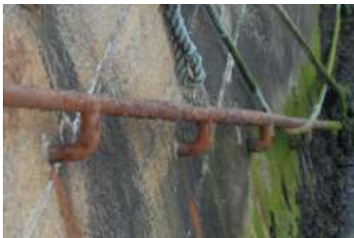
Pitting and General Corrosion Figure 6
