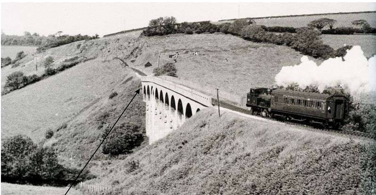
(3) Sunken portion of track
