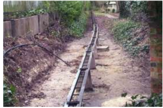
New angle iron supports in place
