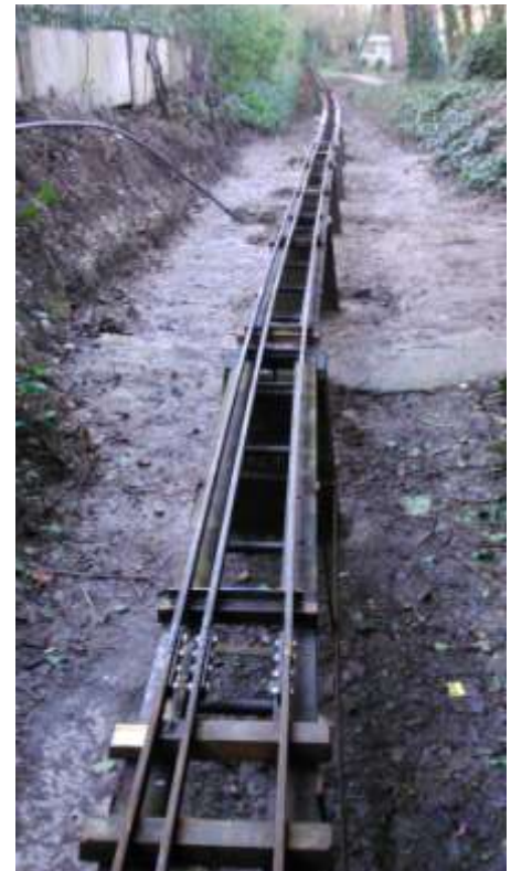
First lengths of new track in place waiting for the curves to be adjusted, ties to be welded and sleepers laid
