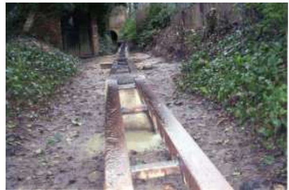
First lengths of new track in place waiting for the curves to be adjusted, ties to be welded and sleepers laid
